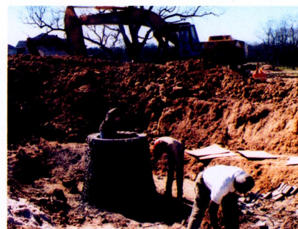
Jimerson crew constructs a manhole that will provide access to the 60-inch storm water line.
