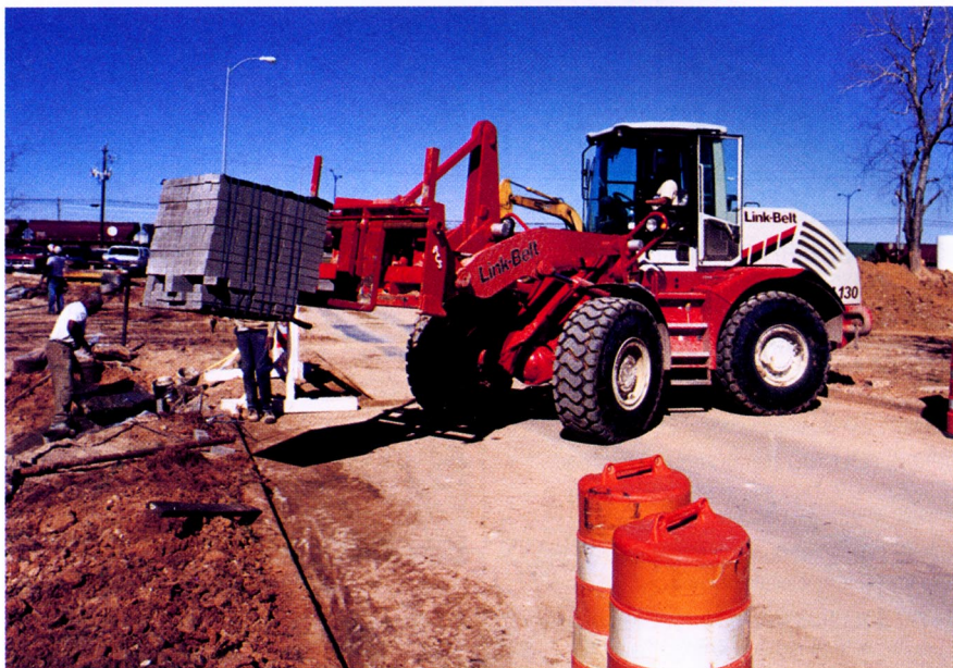
In the toolcarrier application, the new loader transports a pallet of bricks to be laid for a manhole entry.
