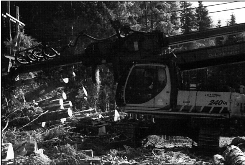
DELIMBING ON THE TOWER SIDE IS ACCOMPLISHED UTILIZING A LINK-BELT 240 LX WITH A PIERCE "DELIMINATOR" MOUNTED ON THE MACHINE.
