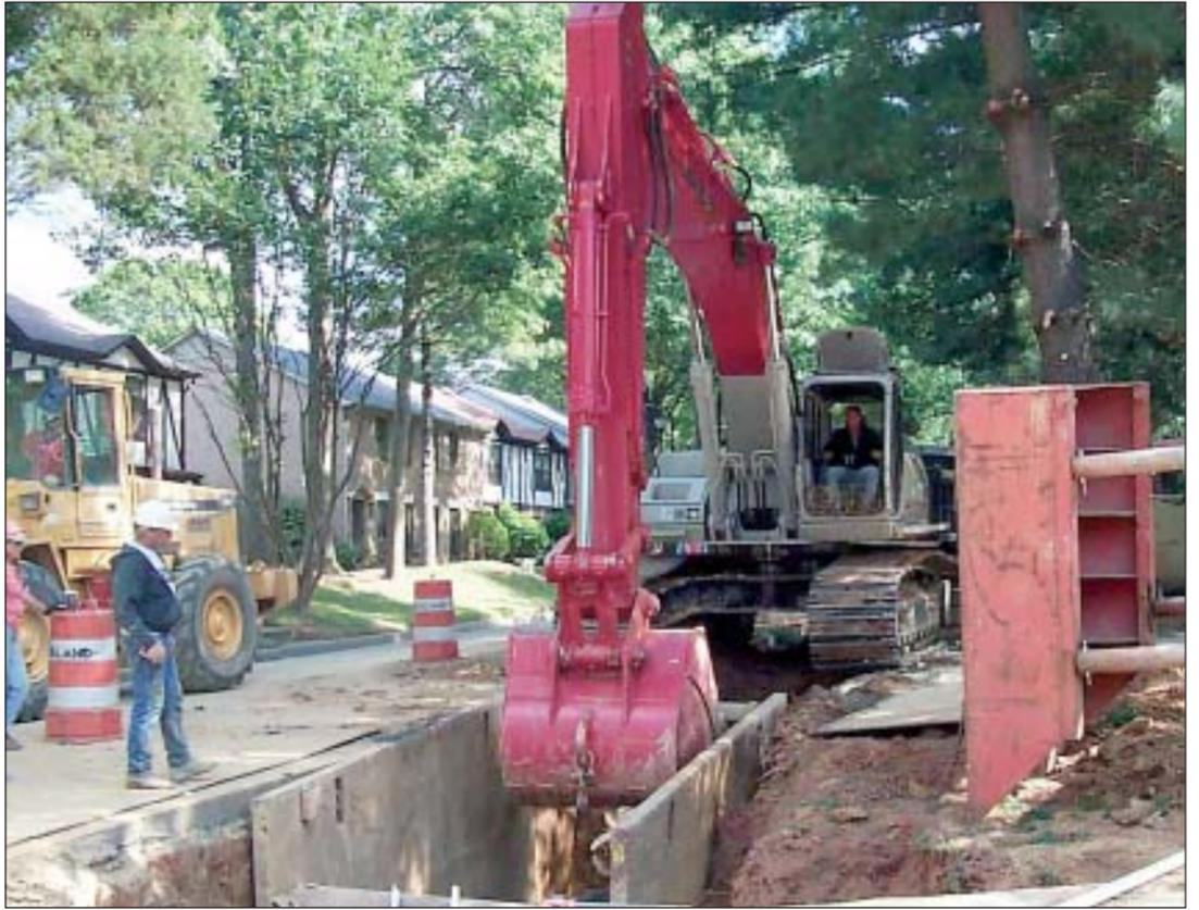
The Link-Belt 460LX excavator, weighing in at 103,000 lbs. (46,720 kgs) is a versatile machine. Here it is setting in the 60-in. (152 cm) pipe.
